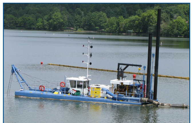
670-42 ft. (12.8 m) dredging a river
